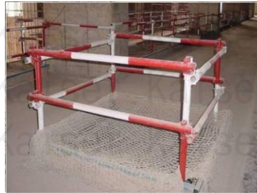
Opening Protection 洞口防护
