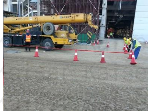
Hoisting Area Fence 吊装区域围护
