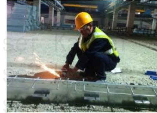
PPE (Cutting Glasses, Ear Plug) 安全护具佩戴 (切割护目镜、耳塞)
