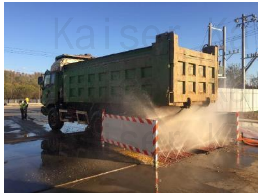
Vehicle Washing 进出车辆冲洗
