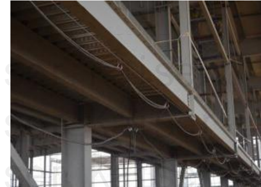
Cable Overhead Installation 电缆临时挂设
