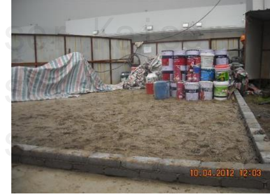
Paint Containment Site 油漆防渗漏堆场
